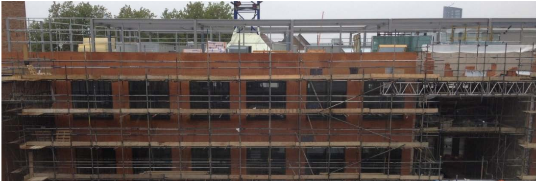
Figure 11: Part of the new Stratford library complex
