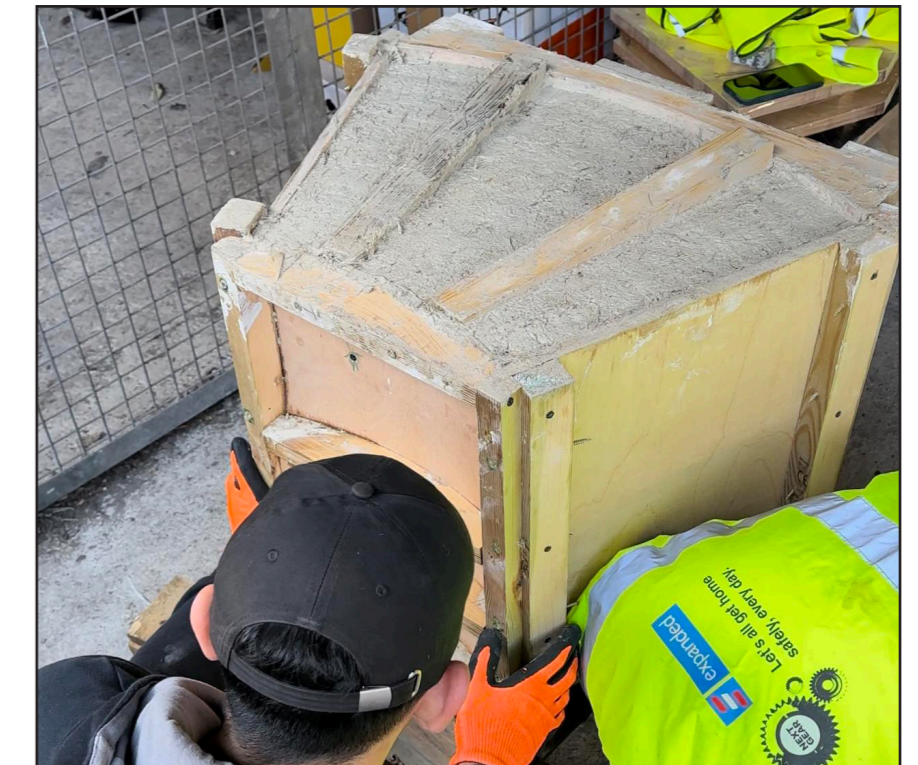
Fig. 92 - UNSCREWING THE WALLS FROM THE BASE
