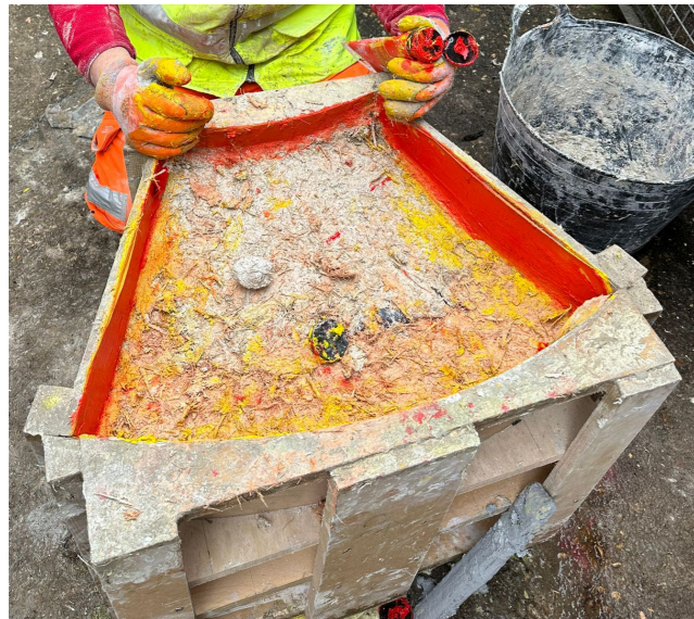
Fig.85 - COATING THE WALLS
