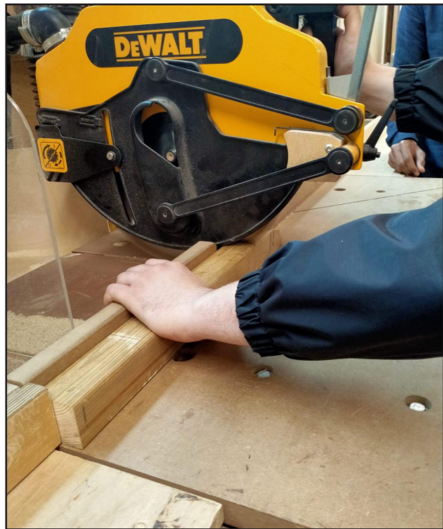
Fig. 62 - CUTTING THE THE BATTENS TO THE RIGHT LENGHT
