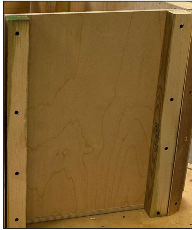
Fig. 61 - SCREWING THE BATTENS INTO THE WALL
