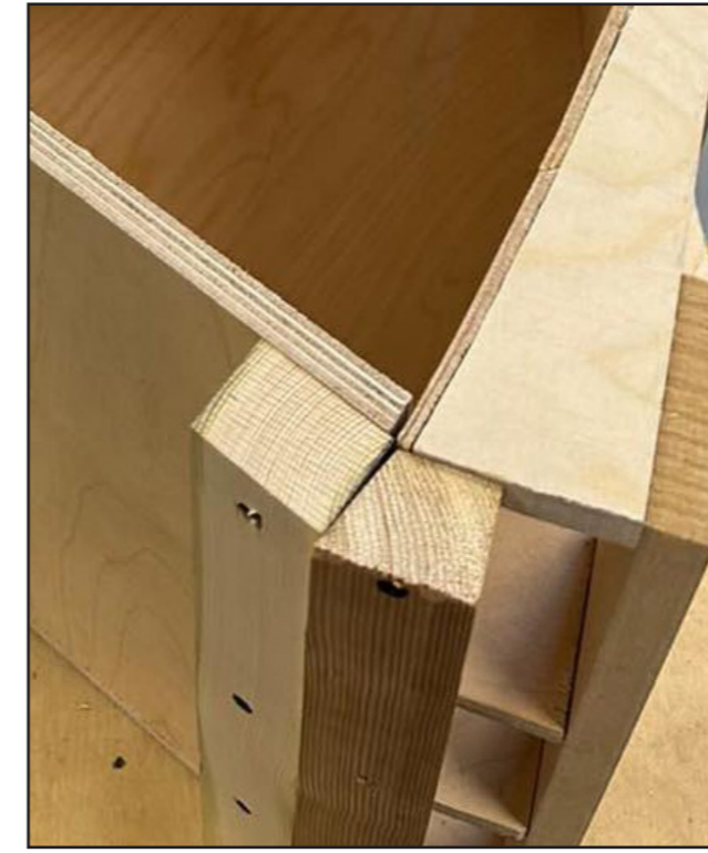
Fig. 64 - A CLOSE-UP OF THE BATTENS ALIGNED
