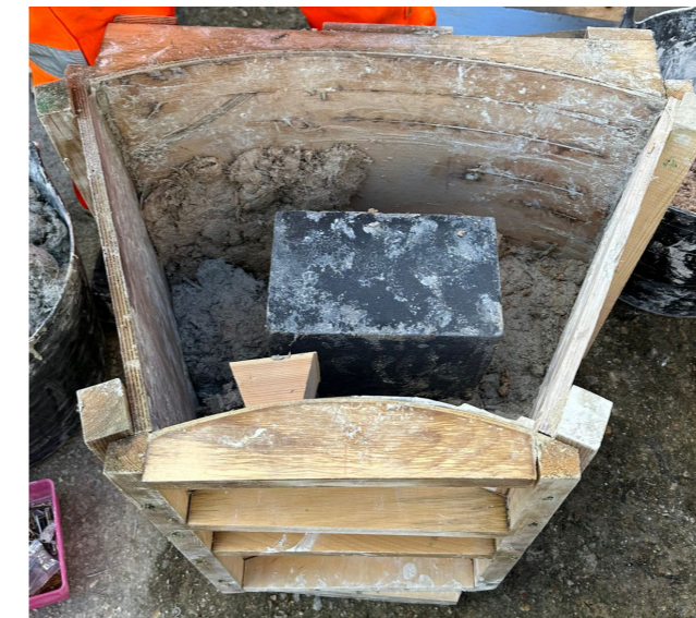
Fig.84 - The void and blocks inside the mould
