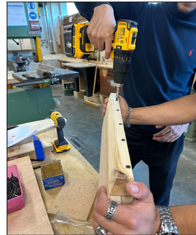
Fig. 65 - SCREWING THE BATTEN INTO THE RIBS
