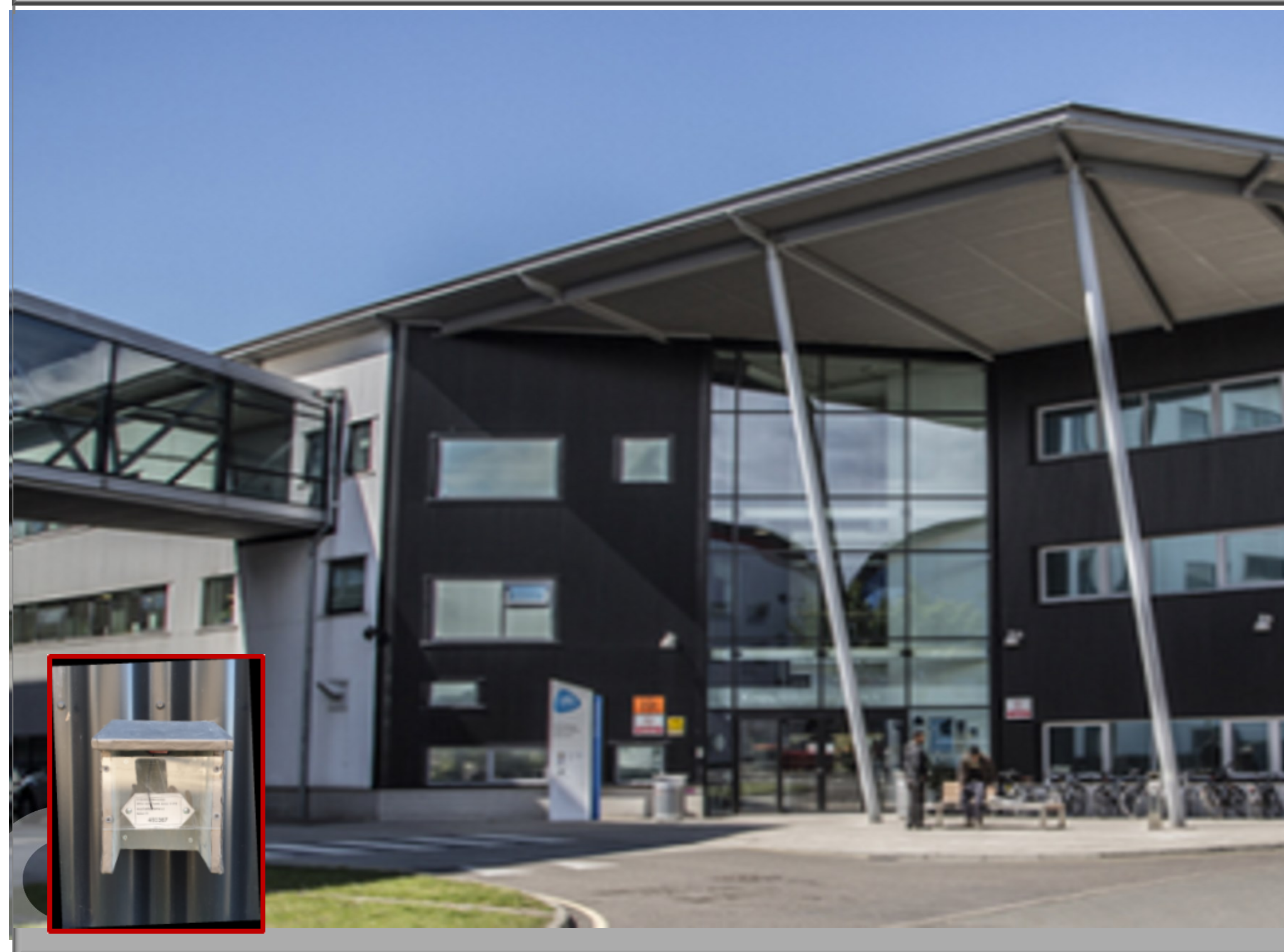
Fig. 1 Knowledge Dock building, UEL, where distributed wireless sensors are installed
