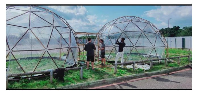
**Pollution Pods on the Green at the University of East London:** The Pollution Pods is an immersive installation made up of five geodesic domes, emulating polluted environments in cities globally. Two of the Pods are currently being erected as part of the MArch 'construction week' and will be on display at Docklands from 27 September until 9 October.
